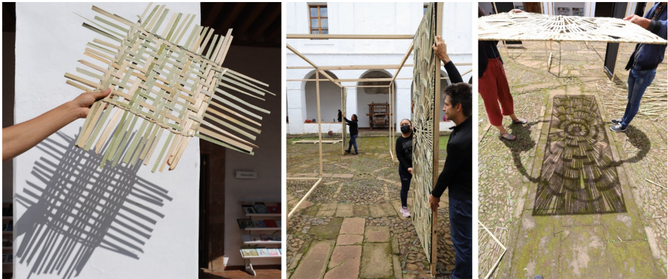
Fig. 6 Prototype experimenting with new weave (left), wooden armature (center), shading test (right). Photos by authors
